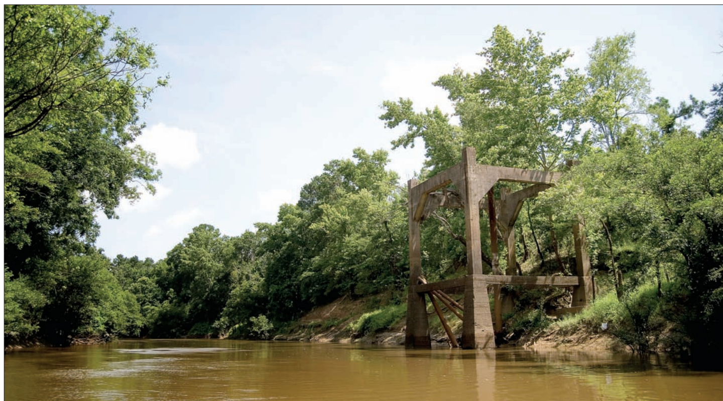
Whatever these giant, concrete pillars were, nature mostly has engulfed them and now owns them for her own uses. The abandoned structures can be found at random spots along the banks of the Sabine River.
